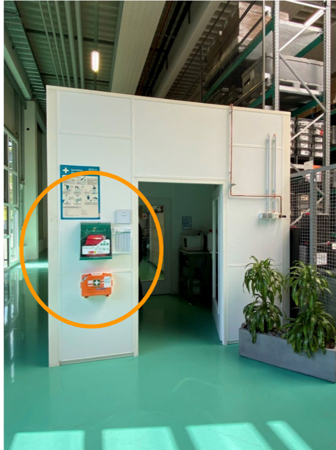
Building 3: on the wall of the service area (near the storage room/other installations)
