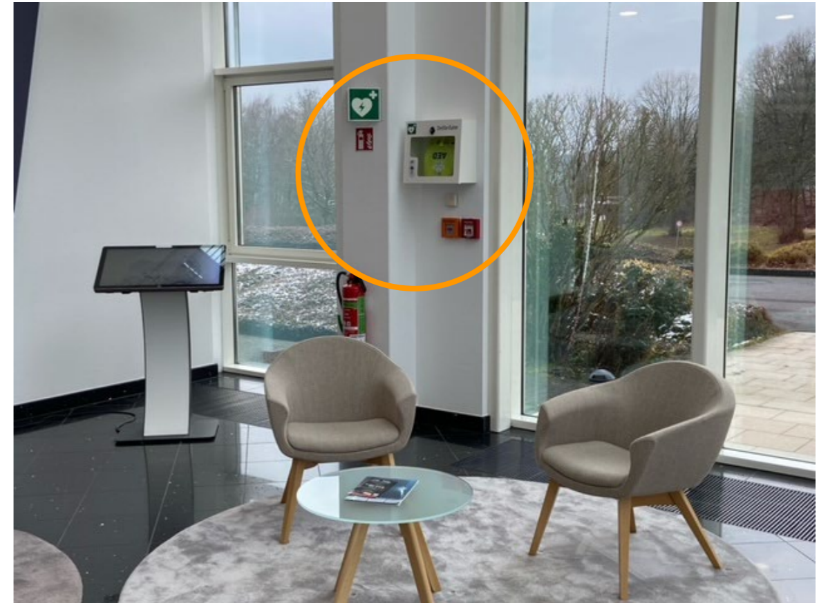
Building 12: in the foyer (outer wall)
